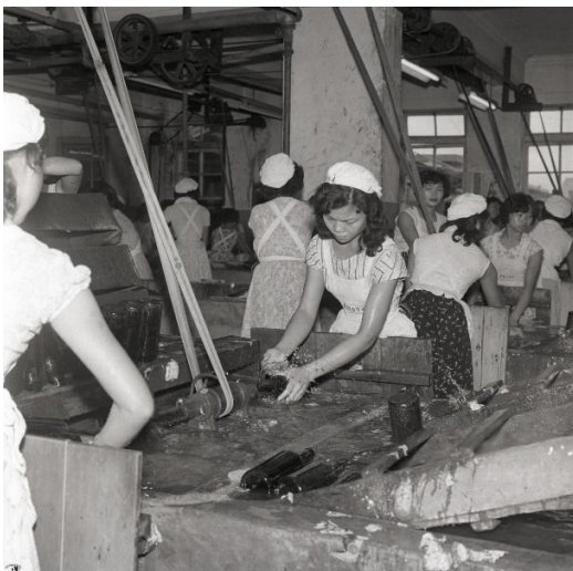
Figure 1. Bottle washing in a beverage factory in Taiwan in the 1960s.
