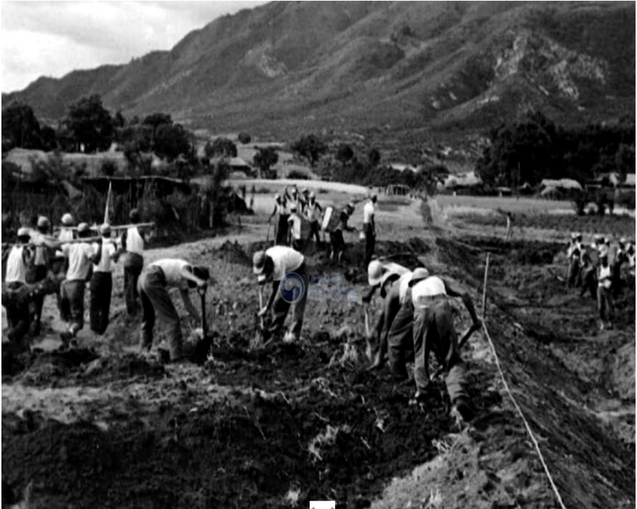
Figure 1. Manual laborers at the Soyonggang Dam Construction Site. Source: "Soyonggang Dam Construction 1 소양강댐건설공사 1," National Archives of Korea, CET0064857.
