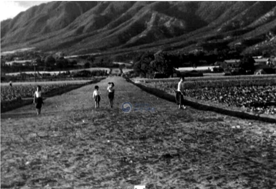
Figure 2. Soyanggang Dam Construction Site. Source: “Soyanggang Dam Construction 2 소양강댐건설공사2,” National Archives of Korea, CET0064857.
